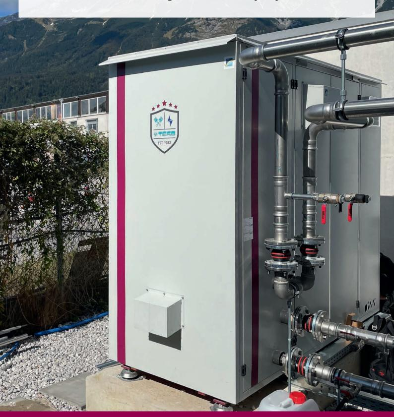
COOLSHIFT CO<sub>2</sub> chillers and heat pumps provide an environmentally friendly and efficient solution for heating and cooling – with maximum energy efficiency. The systems are available in various configurations: chillers as air- or water-cooled versions and heat pumps in air/water, water/water, or air/air designs. They are offered in sizes M, L, and XL and can be installed both indoors and outdoors. The COOLSHIFT series covers a heating or cooling demand of up to 4 megawatts.
