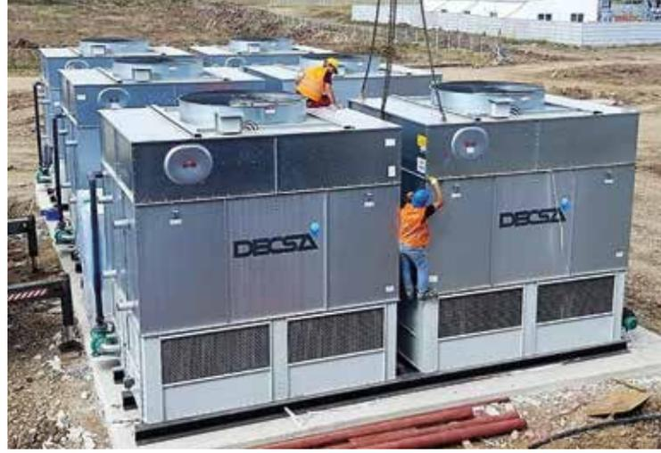
air-cooled condensers often reach their limits so that condensing temperatures can reach  $> +48$  °C. By using the DECSA evaporative condenser, it is ensured that the condensing temperature does not exceed  $+33$  °C, even when outside air temperatures are high.
