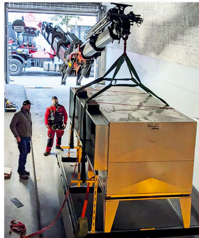
The gas cooler was installed almost horizontally using a loading crane. Copyright rights are held by KOCH – Kälteanlagenbau GmbH.
